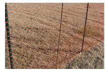
Weaving rebar through the grid of the fence and driving it into the ground between two T-post can help increase the strength of the fence.
