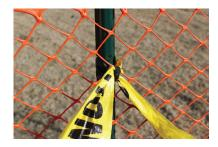
If zip ties are not available you can use Presco Barricade tape or Roll Flagging as a way to secure the fence to the posts.
