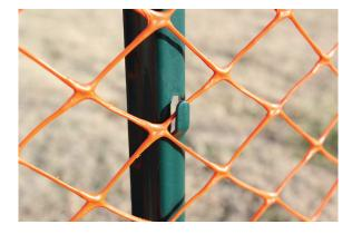
Be sure to utilize the "teeth" of the T-post keep the Safety Barrier Fence from sliding down the post. This will help secure the fence and improve the longevity of the fence.
