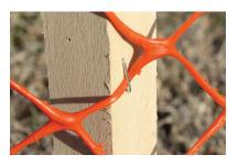
if T-posts are not available and landscaping stakes are used staples, in addition to zip ties, can be used to secure the fence to the stake.
